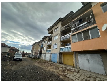
MFB 1 - there are three sections in the building: The three sections have 3 floors each. Total built-up area for the building - 1 794 m 2
